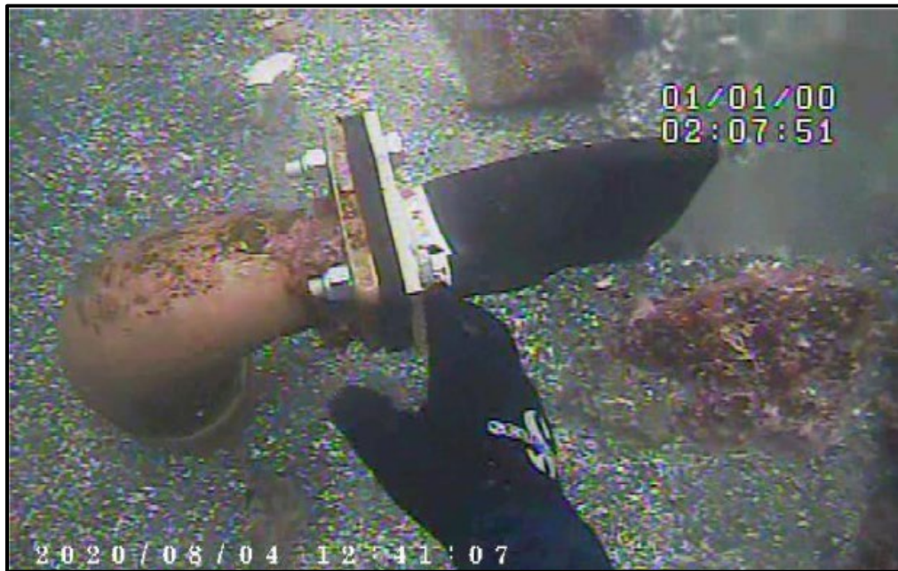
Figure 4-2. A Diffuser Port with TideFlex Check Valve.
