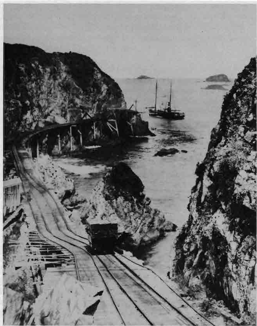
Steam schooner Whitesboro loading at L. E. White Company's wire chute at Greenwood.
