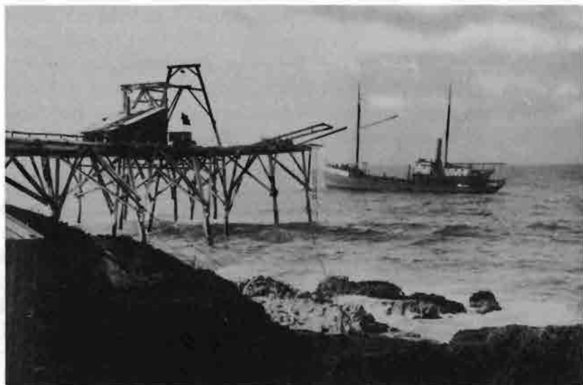
Steam schooner National City loading split ties at the Union Lumber Company's wire chute at Cleone.
