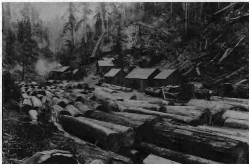
Log drive. In the summer thousands of logs were rolled into stream beds. Winter freshets floated them down to the sawmills, and sometimes—out to sea.
