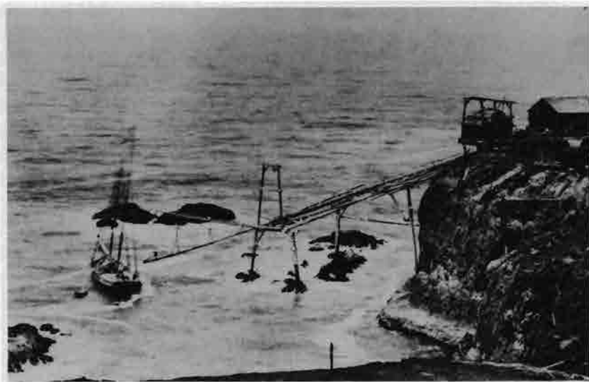
Newport Chute. By means of a wooden chute, lumber from Stewart, Hunter & Johnson's mill was here loaded aboard little lumber schooners.
