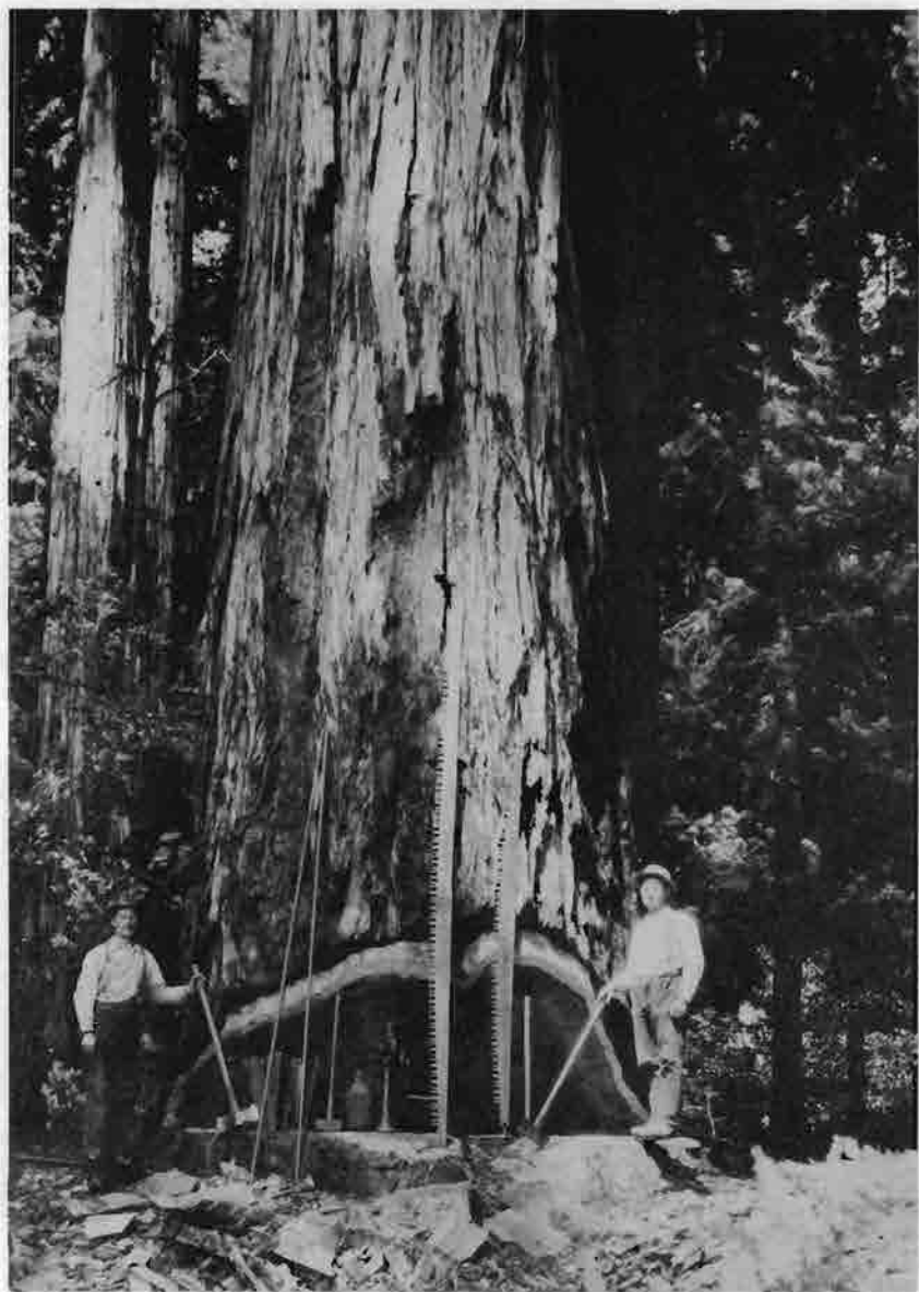
Before the adaption of power saws to the falling of large timber, choppers spent many hours "putting in the undercut."
