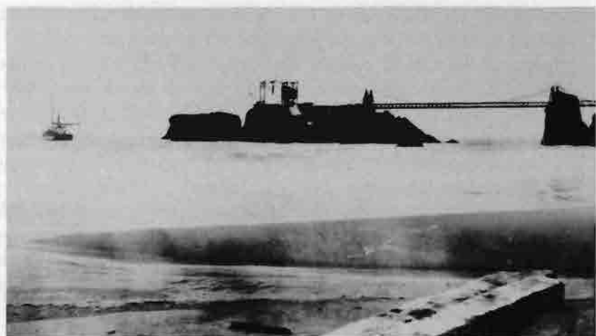
Suspension bridge to the Island at Rockport where wire chute was located.
