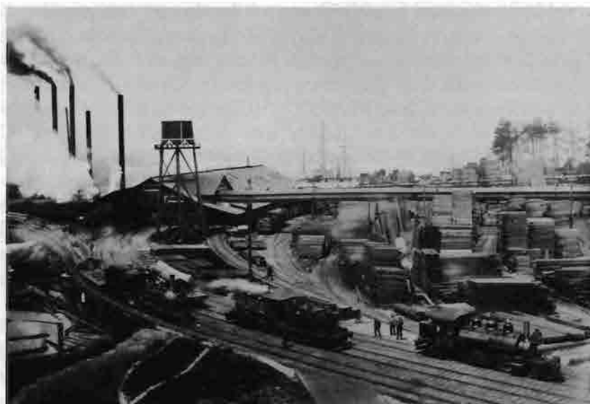
Union Lumber Company's Fort Bragg plant in 1910. Badly damaged by earthquake and fire in 1906, it was rebuilt and enlarged.
