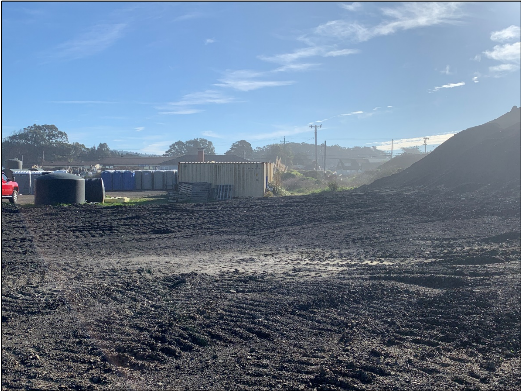
Southern property line and material pile from Geo Agg
