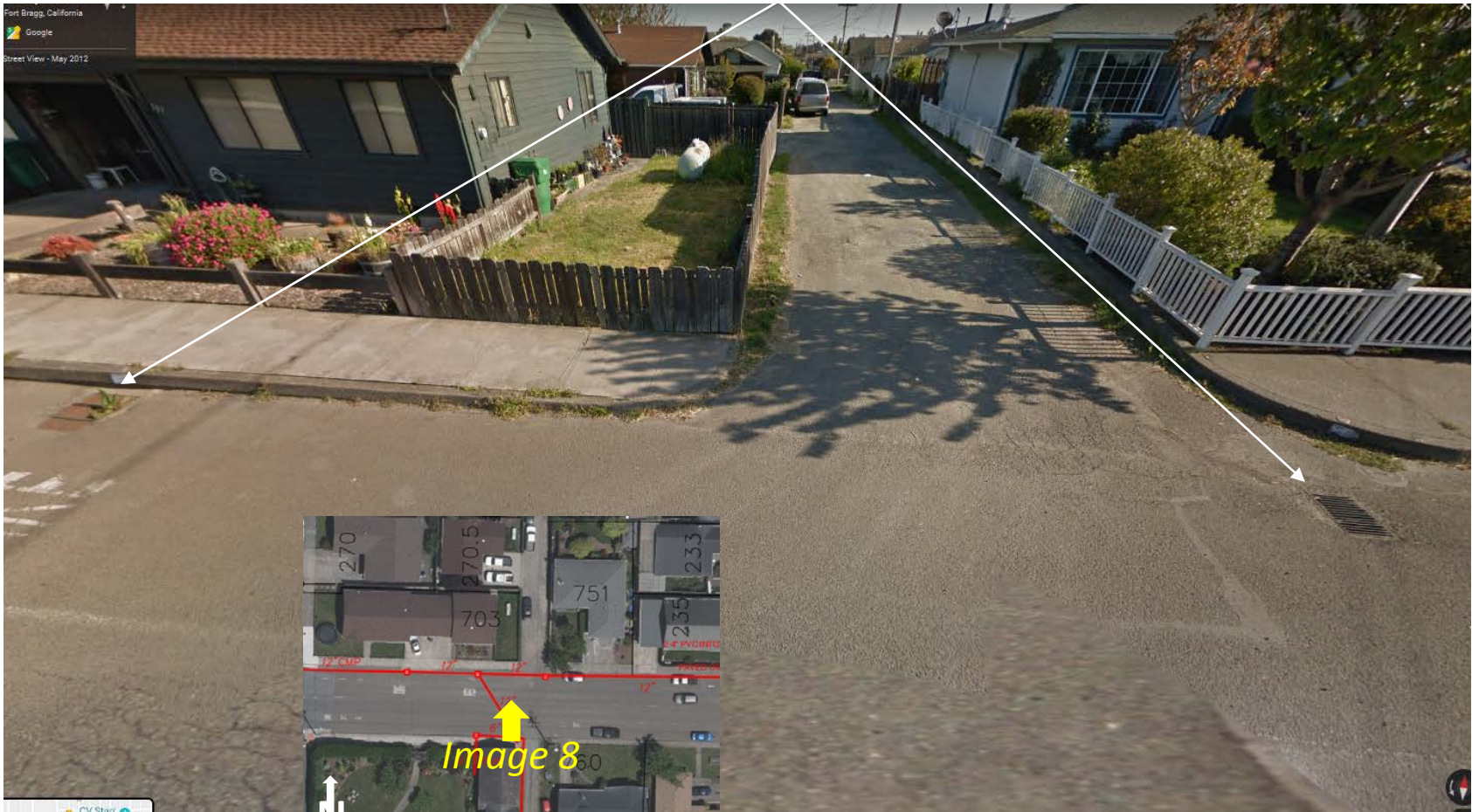
Image 8 – Inlets on north side of Maple at alley
