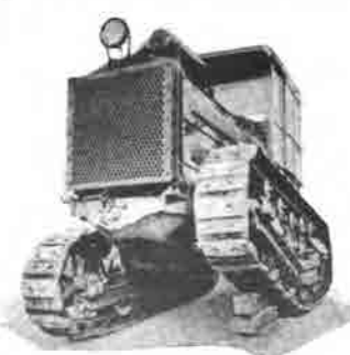
SHOWING TRACK ACTION CATERPILLAR 10 TON
