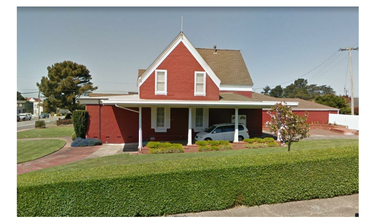
SITE PHOTO - SOUTH
