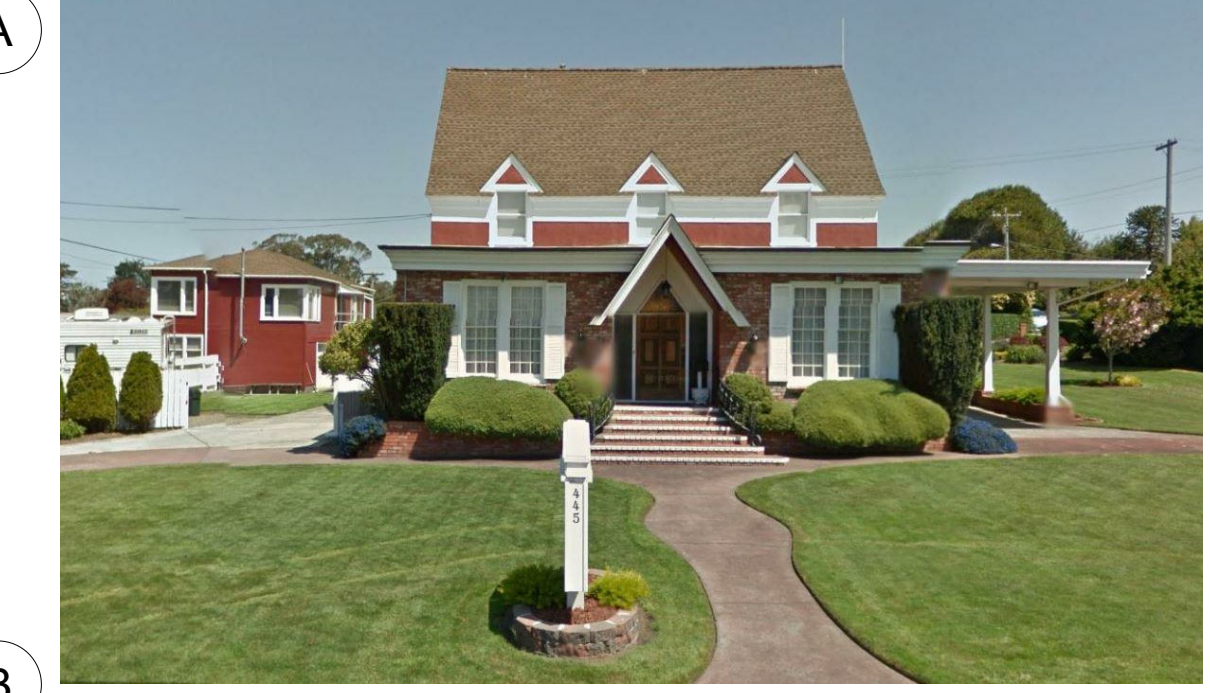
SITE PHOTO - WEST
