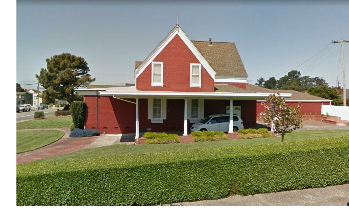
SITE PHOTO - SOUTH
