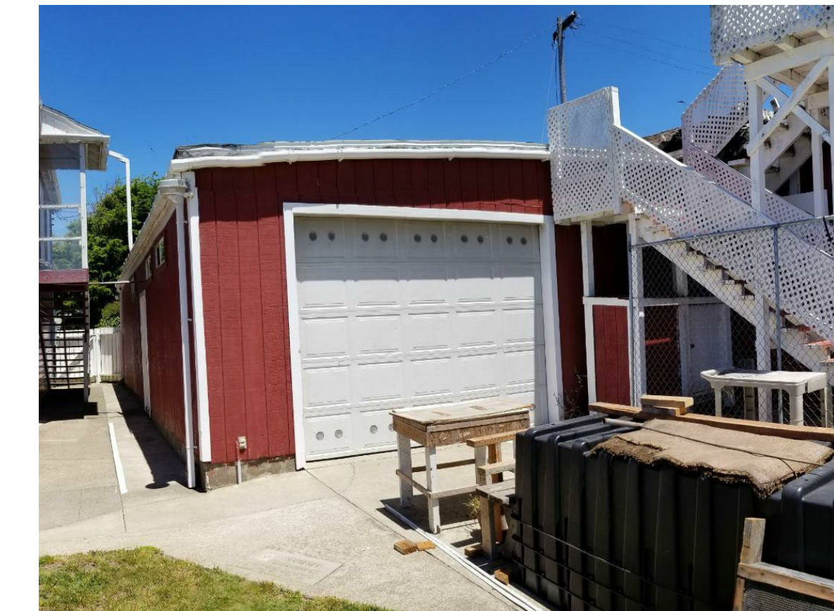
SITE PHOTO - GARAGE SOUTH
