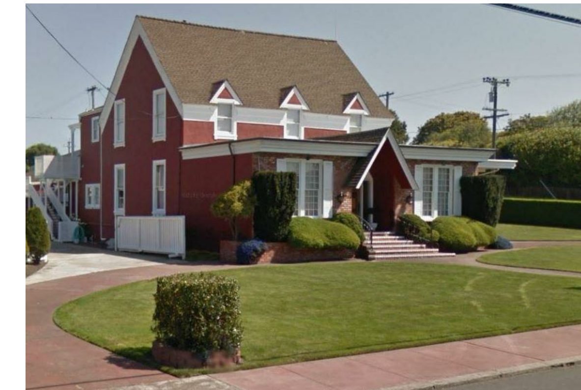
SITE PHOTO - WEST
