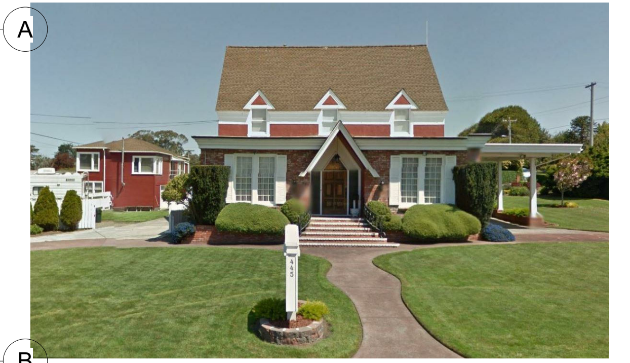
SITE PHOTO - WEST
