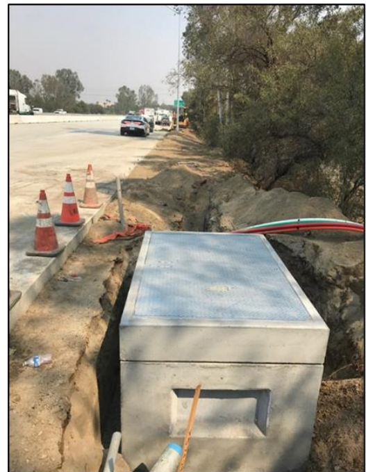
Figure 7. Vault Installation
