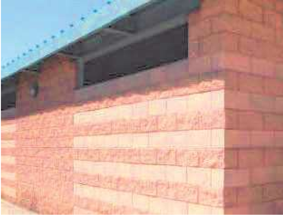
Figure 2. Example showing both smooth and splitface concrete blocks
