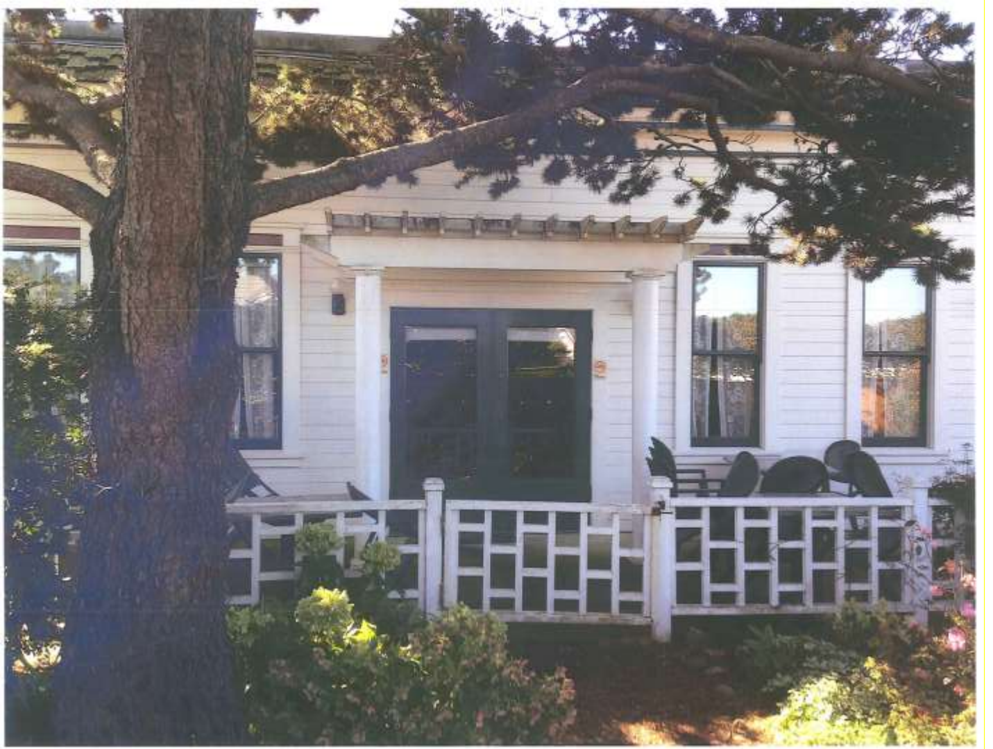
Attachment 4: Existing Patio from Front
