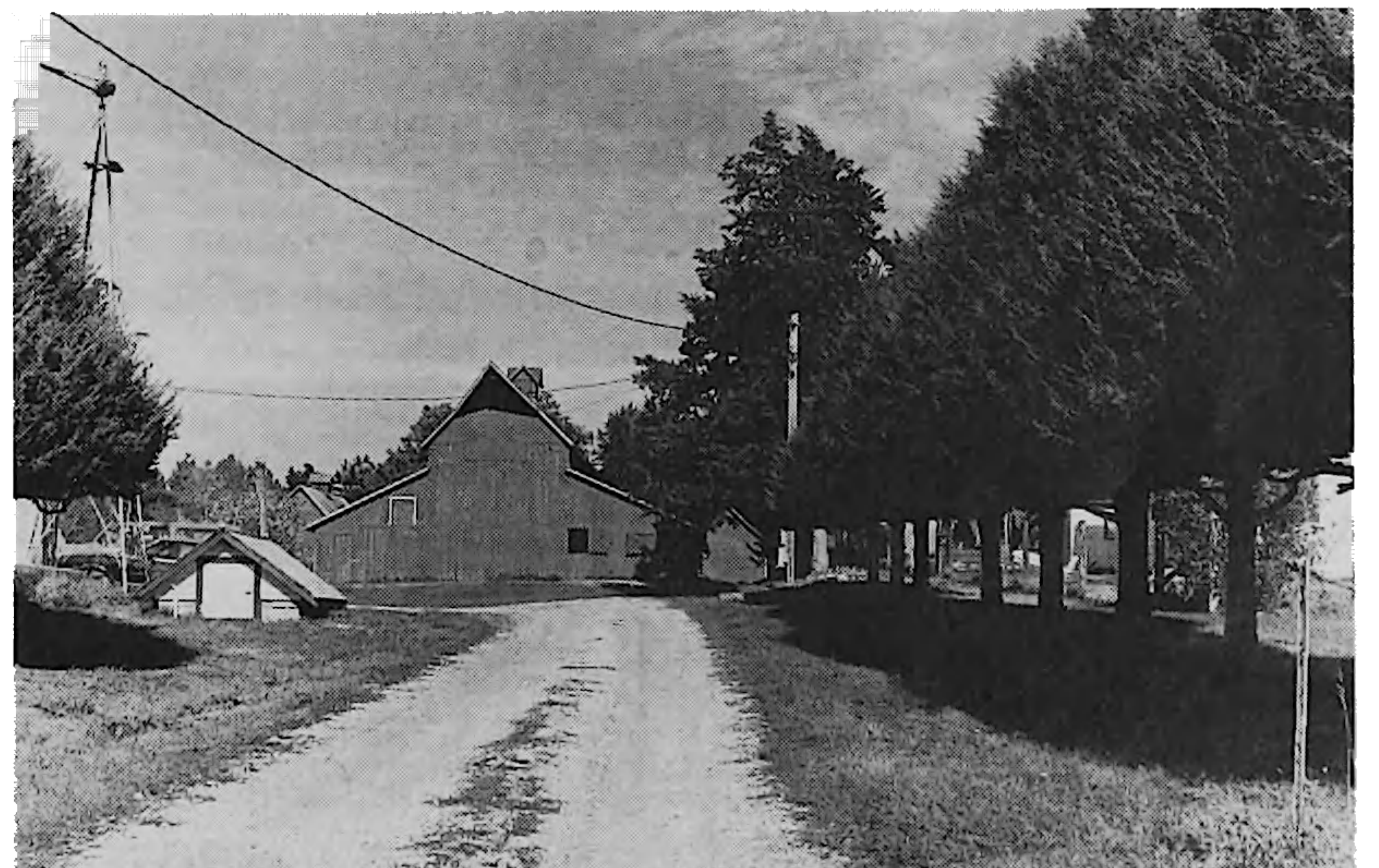
Figures 22 and 23: The plan for the Kehlbeck Farmstead, located in Cass County in Southeastern Nebraska, illustrates a well-planned, and aesthetically arranged general farm complex of the twentieth century. The farmstead is composed of 23 contributing and 5 non-contributing resources. Integrity was judged uniformly high because many character-defining resources were present and the visual and spatial relationships intact. Note the varied graphic techniques used to document a variety of fence types, and, the key to photographs illustrating the various landscape features and spatial relationships. The photograph above, labeled #3 on the farmstead, is looking north along the farm lane alley. (courtesy National Register Files)
