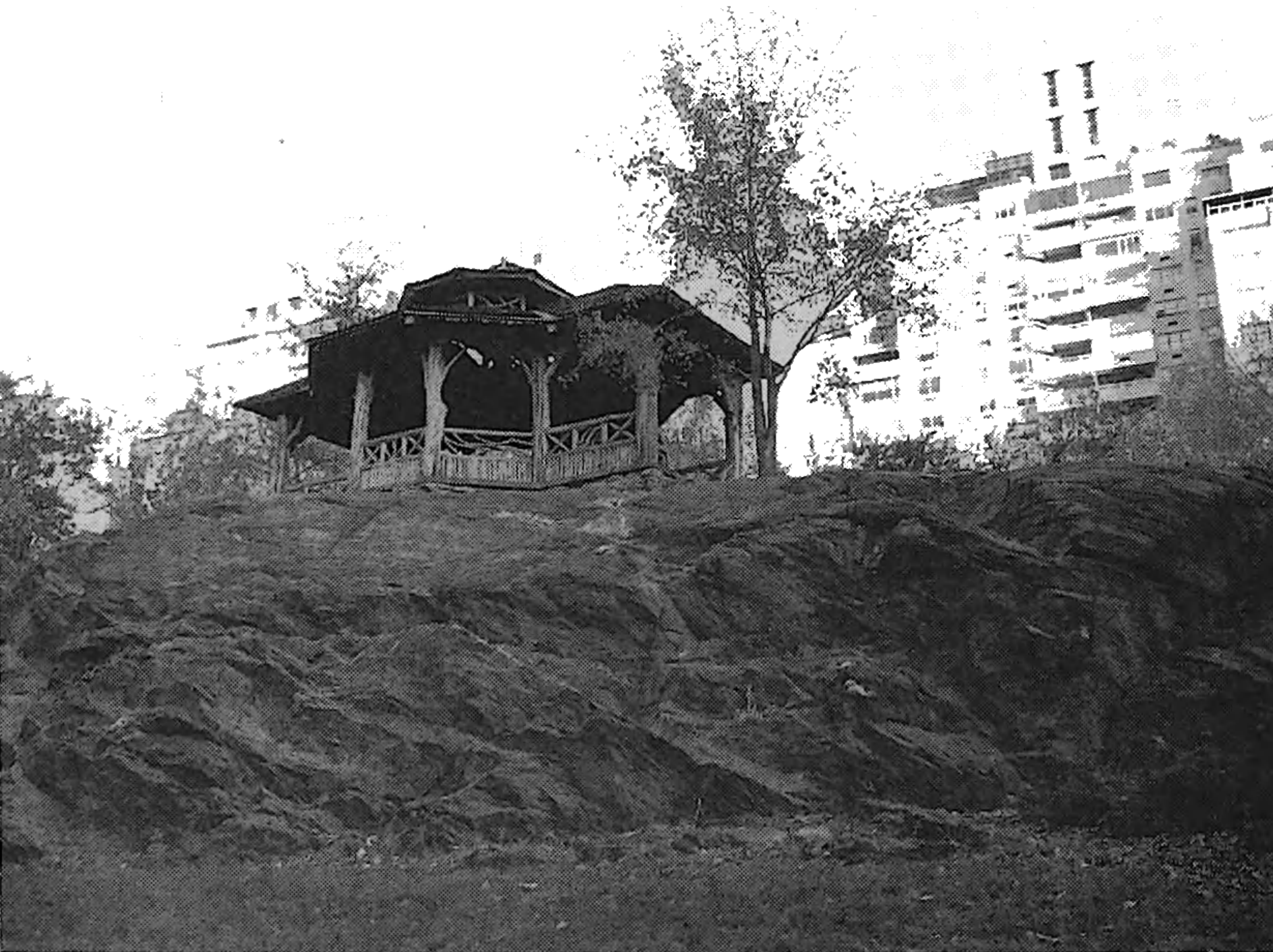
Figure 35-37: Central Park has developed an in-house historic preservation crew to undertake small projects. A specialized crew has been trained to specifically repair and rebuild rustic furnishings. As illustrated, the restoration of the Dene rustic shelter was achieved by constructing it in the Ramble compound, moving in-place opposite 67th street and completed. (courtesy Central Park Conservancy)
