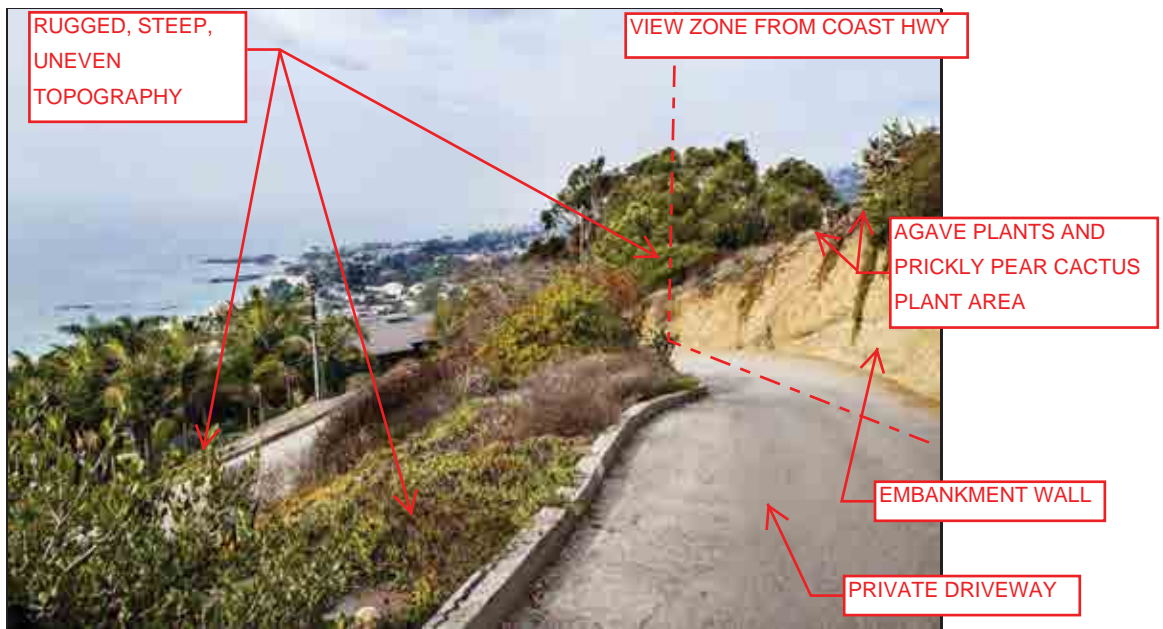
Circulation Features, Topographic Characteristics, Vegetation Features, Views and Setting, 31162, 31164 Ceanothus Drive
