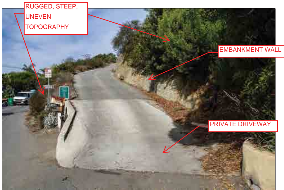
Circulation Features, 31204 Ceanothus Drive
