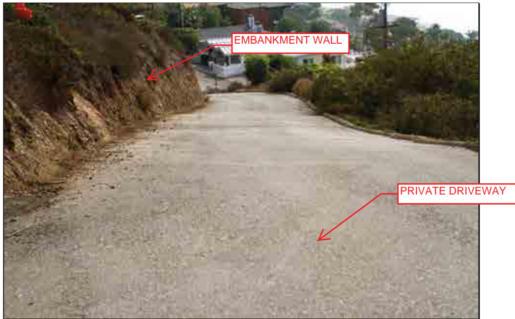
Circulation Features (embankment wall and driveway detail), 31164 and 31204 Ceanothus Drive
